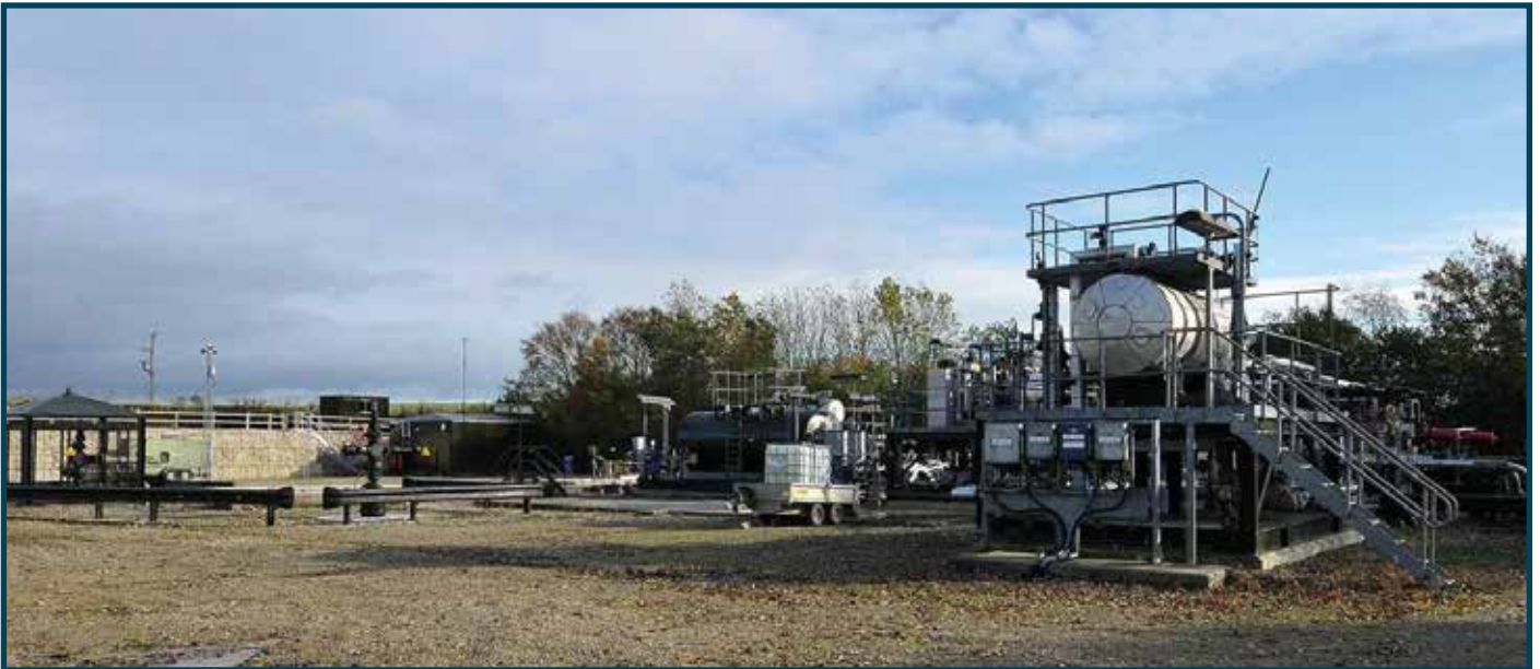
The existing brownfield site at Kirby Misperton
